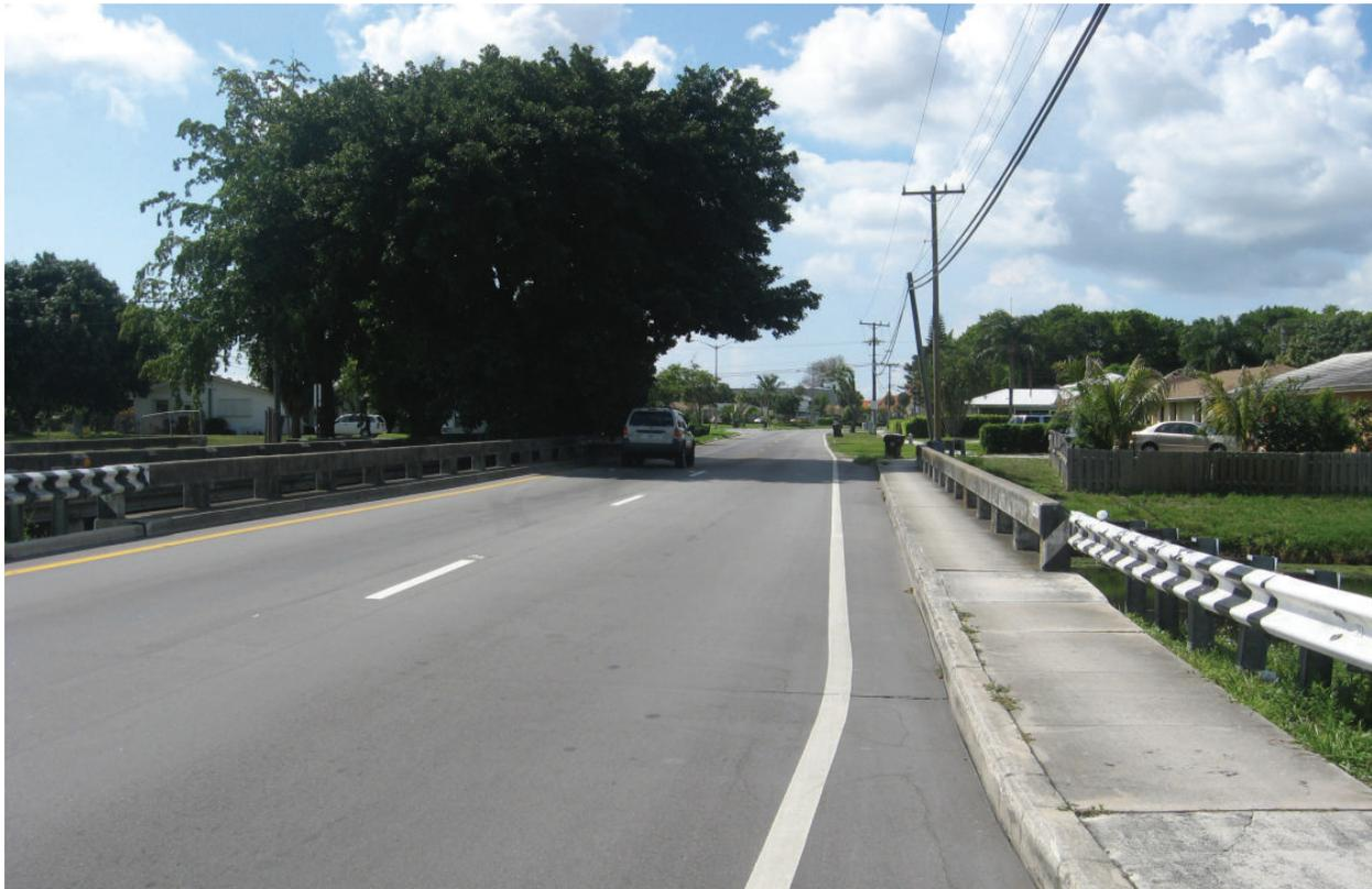
Figure 5A.6: Branches from a tree in the median encroach on the inside lanes of the bridge south of 45<sup>th</sup> Street.
