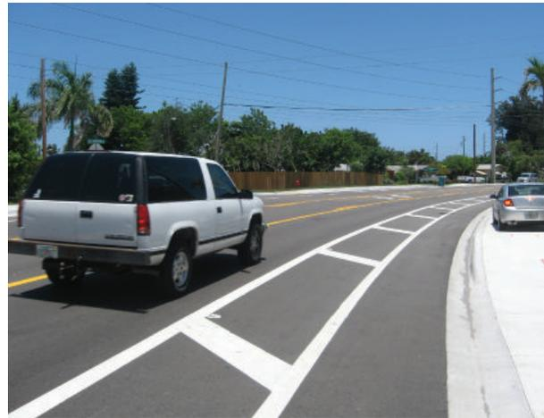
Figure 5A.30: Buffered bike lane through curve on Old Boynton Road
