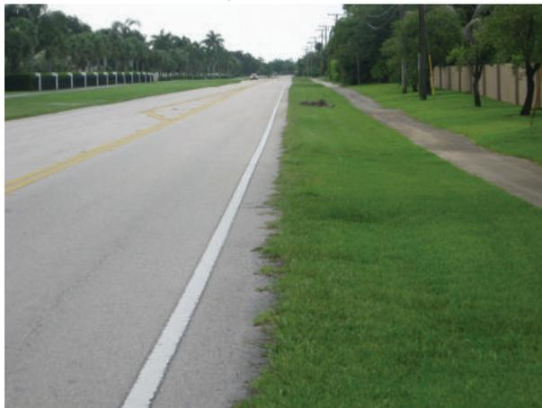
Figure 5A. 3: Shoulder widths are variable and have been encroached by vegetation
