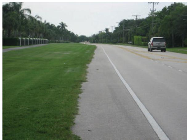
Figure 5A.2: Shoulder widths are variable and have been encroached by vegetation
