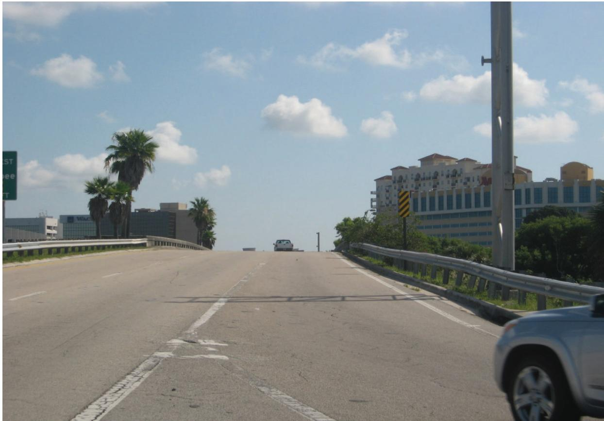
Figure 5A.8: Vehicles using the acceleration lane on the Okeechobee Boulevard overpass merge quickly as the lane is taken away on the far side of the bridge
